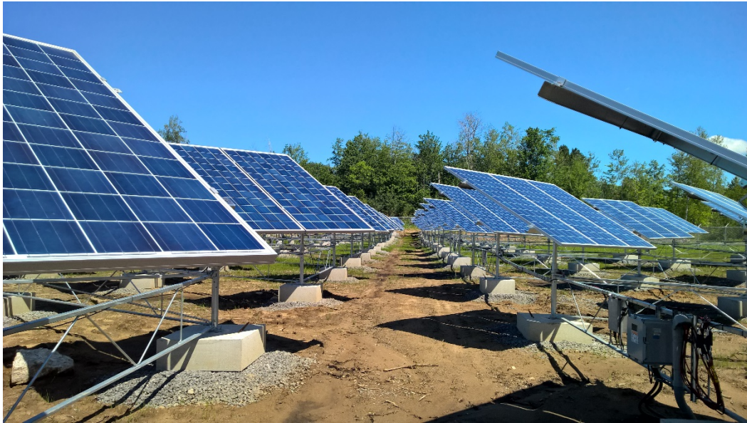
Figure 8: One of the Sundance Projects utilizing Morgan Solar Savanna trackers.
